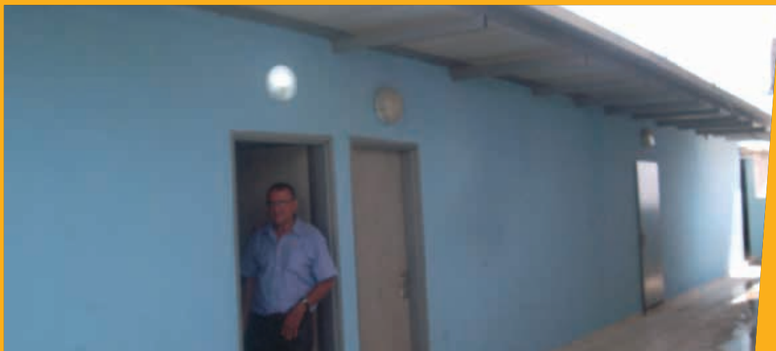
The conclusion of the project for the renovation and rehabilitation of Al-Esawyyah Club.
