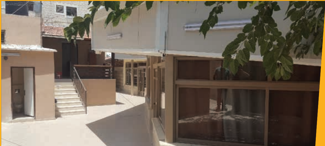
The conclusion of the project for the comprehensive renovation and rehabilitation of Silwan Sports Club.
